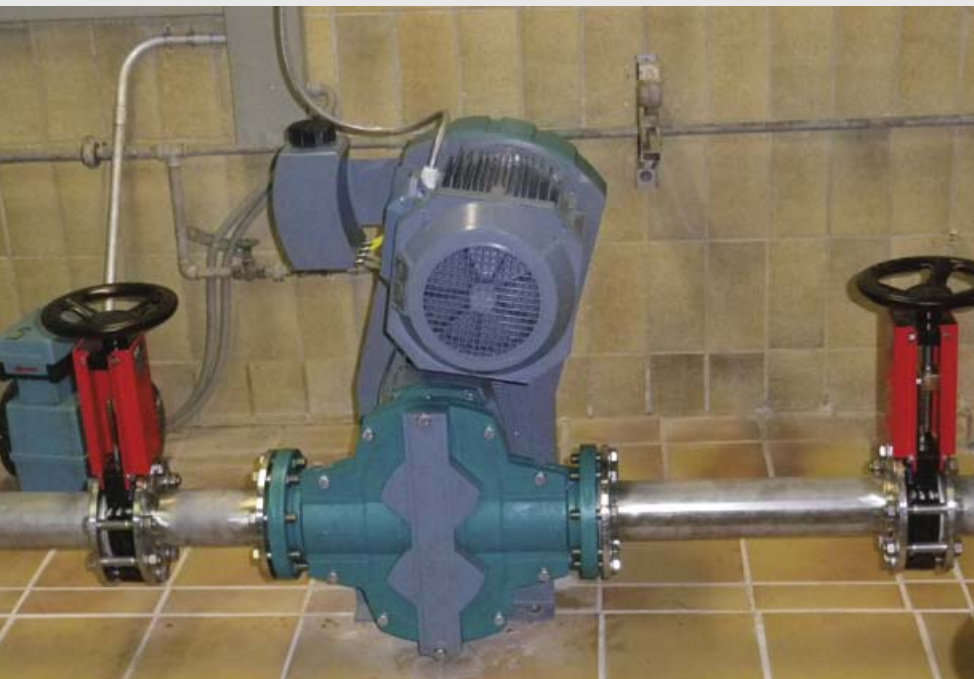
Used in a wastewater treatment plant, the TORNADO® T2 pumps sludge with 2% solid content at a capacity up to 18 m 3 /h against a pressure up to 2 bar.
